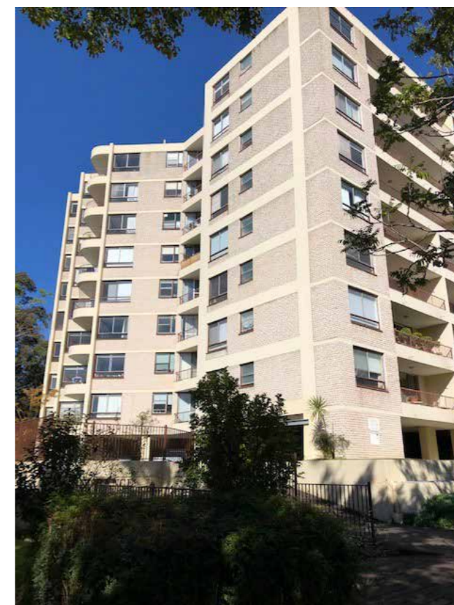
Figure 25 Detail east elevation Sutherland Gardens at 8-12 Sutherland Road
