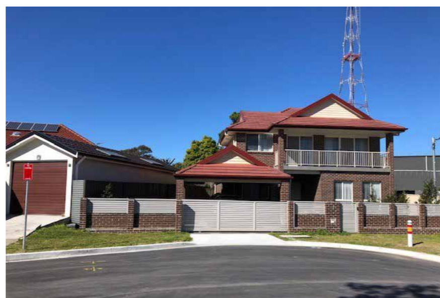
Figure 16 Streetscape character of Berkely Court on the eastern side of the rail corridor at 2 Berkely Court
