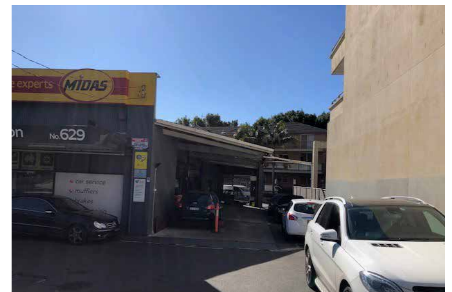
Figure 11 South-west elevation adjoining the RFB on Hammond Lane, corner of Gordon Avenue
