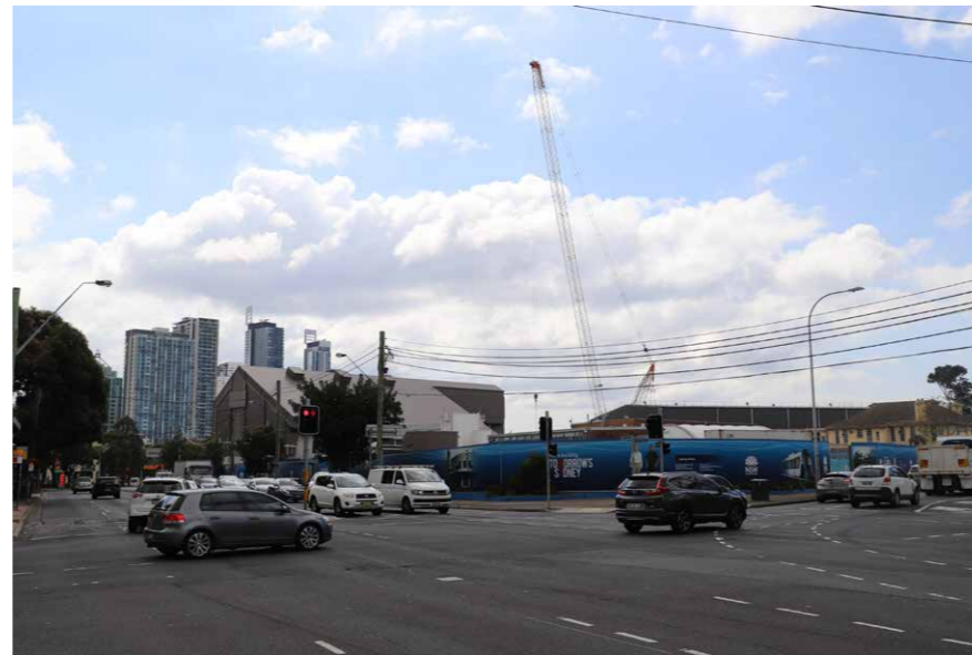
Figure 57 From the south-west corner of Mowbray Road and the Pacific Highway
