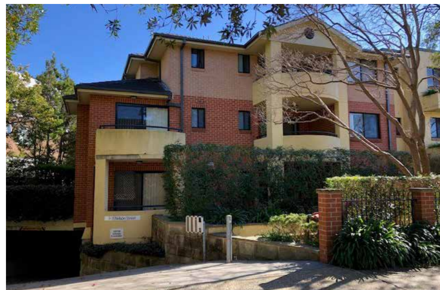
Figure 3 Detail view of the south elevation of 9-11 Nelson Street
