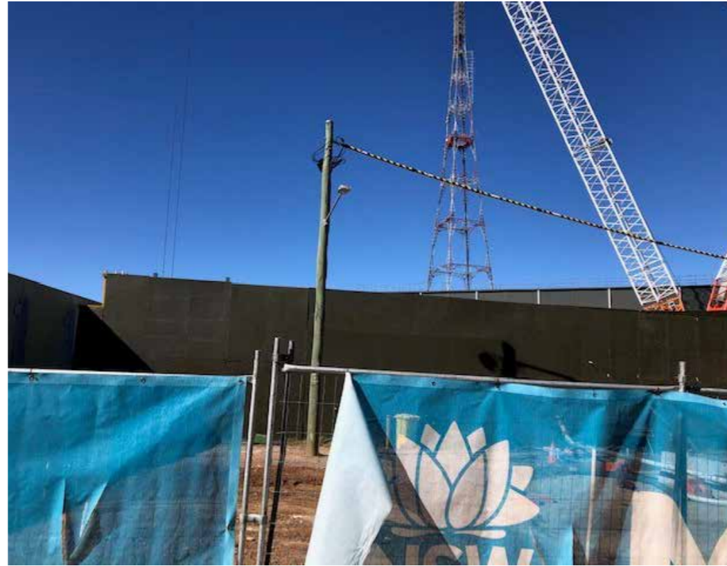
Figure 13 Views looking south from the front elevation of 9-11 Nelson Street
