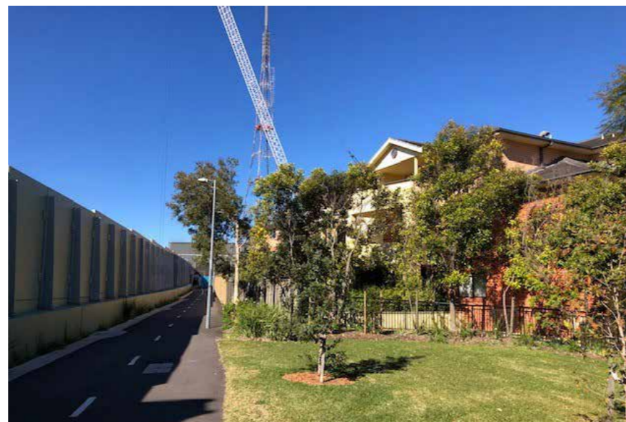
Figure 4 View looking south toward the south-east elevation of 9-11 Nelson Street
