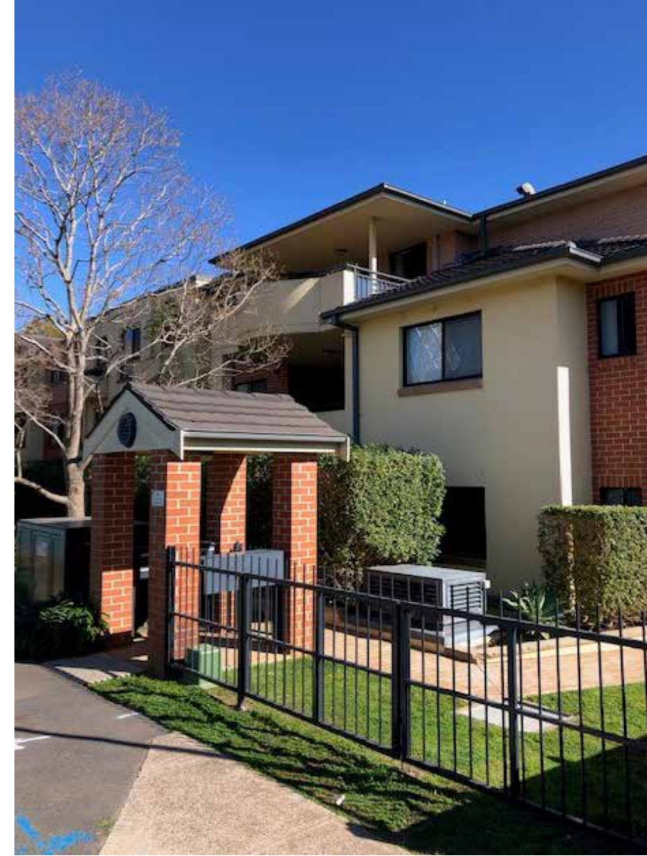
Figure 6 Detail view of the south-east corner of 9-11 Nelson Street
