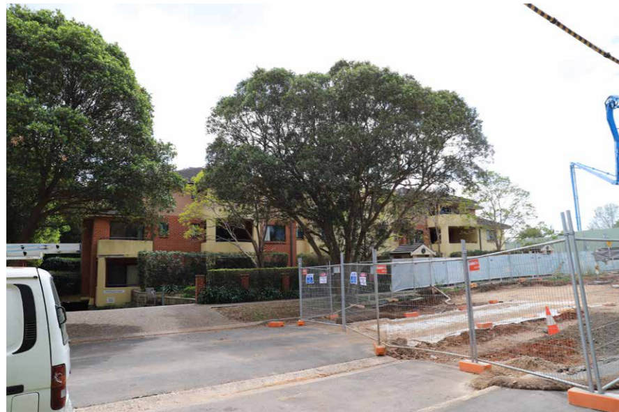
Figure 55 Site detail from Nelson Street
